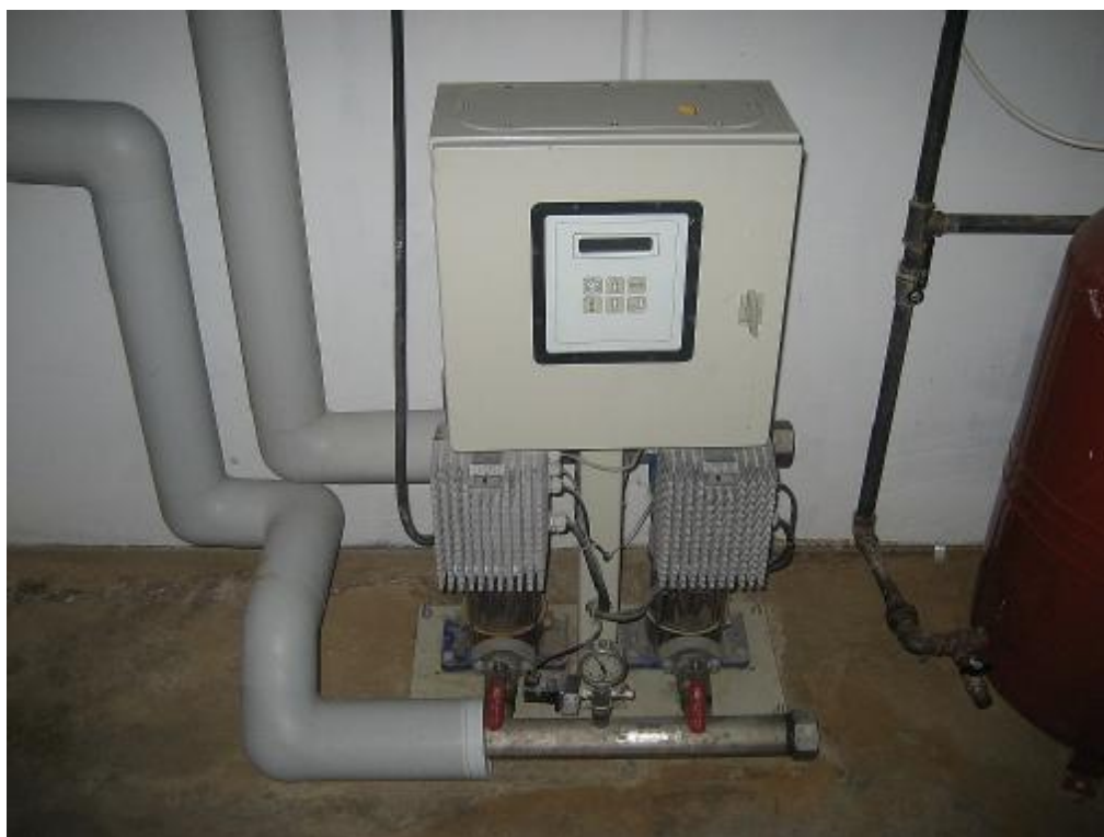
Pumpe i drift
